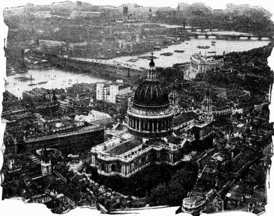
TYPICALLY LONDON. This aerial view of part of the great metropolis with St. Paul's, which is symbolic of London, in the foreground shows the Thames winding towards Westminster. Twice this week London is featured in the programmes.
